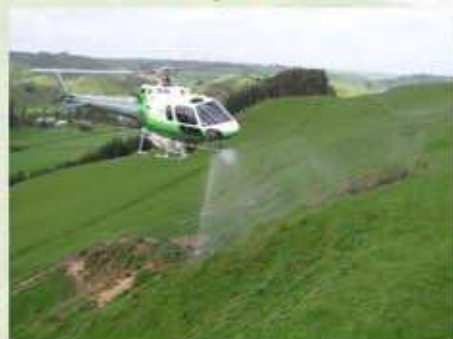
helicopter hydroseeding
