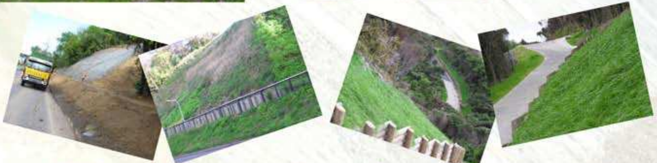
Swale drain treated with Evergreen BioMat bonded fibre matrix
