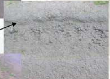
Close up view of swale drain showing covering of Evergreen BioMat bonded fibre matrix
