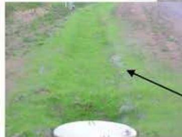
Close up view of swale drain showing covering of Evergreen BioMat bonded fibre matrix
