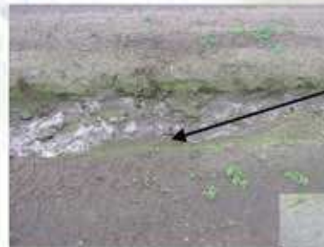
Close up view of swale drain showing covering of Evergreen BioMat bonded fibre matrix
